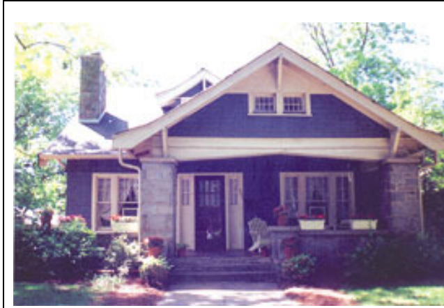
Acceptable: Large porch, acceptable stone columns, inviting entry-way and lots of character.
