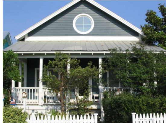
Unacceptable: Columns too small, otherwise acceptable.
