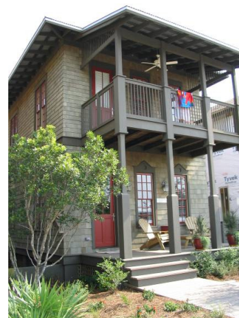
Unacceptable: Porch too shallow otherwise, siding, deep roof overhangs and column design acceptable.
