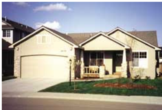
Unacceptable: Front porch too small, not constructed on raised foundation and garage not setback from front elevation.
