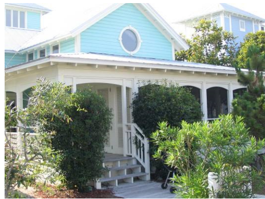
Unacceptable: Columns too narrow, otherwise acceptable. Note good use of arches between columns.
