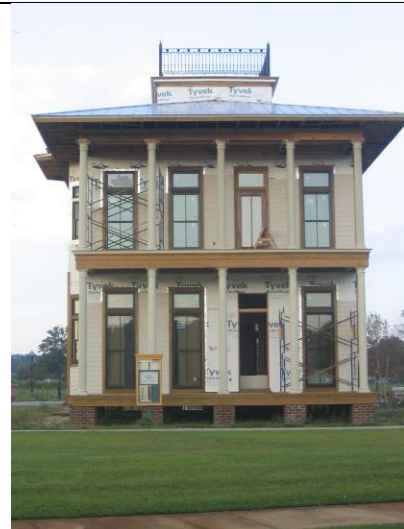
Unacceptable: Porches too shallow, however, roof over hangs, column design, foundation design, color scheme and height are excellent.
