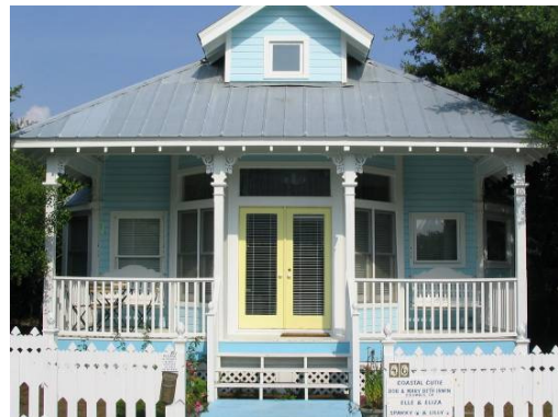
Acceptable: Lots of character, raised foundation and large front porch.
