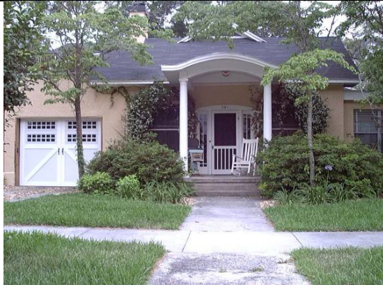
Unacceptable: Although house has significant character, the porch is not large enough. Please note excellent garage door detailing.
