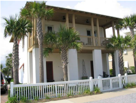
Unacceptable: Insufficient foundation height, unwelcoming front entry-way and porch too shallow.
