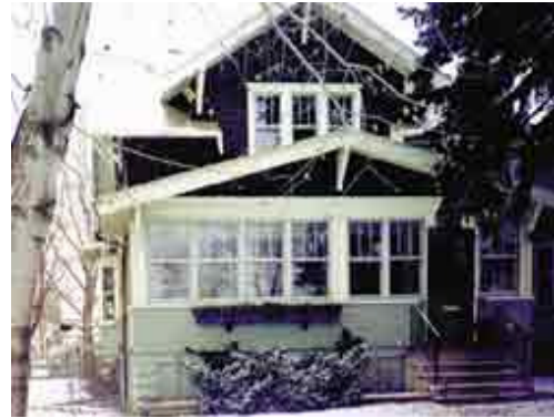
Unacceptable: Enclosed front porch otherwise has interesting rooflines, deep roof overhangs and brackets.
