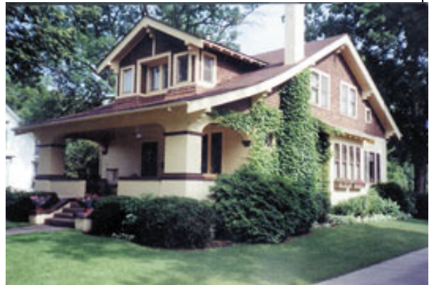
Acceptable: Large porch and plenty of character, good use of climbing vegetation, however color scheme is suspect.
