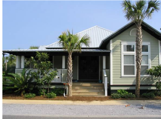
Acceptable: Porch covers at least 50% of front elevation, utilizes raised foundation, and has acceptable color scheme and roofline.
