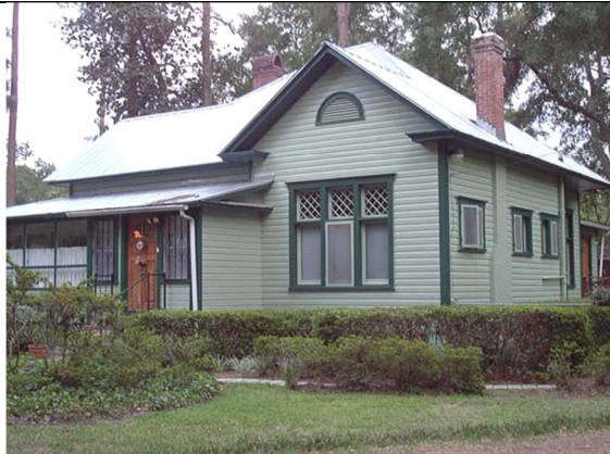
Unacceptable: Front porch enclosed, iron handrails, however roofline, window casing and color scheme acceptable.
