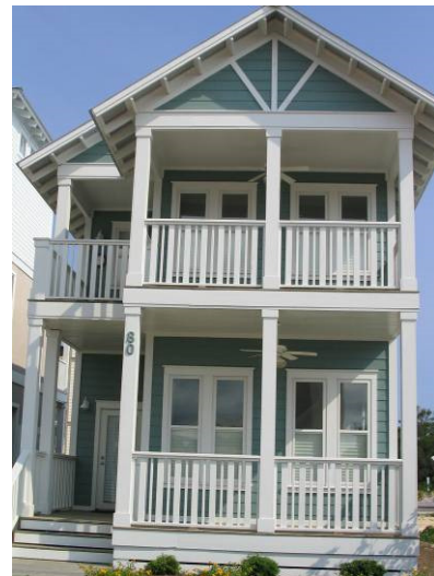
Unacceptable: Entry-way uninviting and porch too shallow otherwise acceptable.
