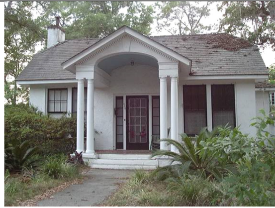
Unacceptable: Although this house has significant character and good column detailing, the front porch is too small. Please note acceptable roofline.
