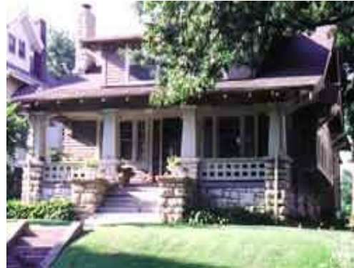
Acceptable: Lots of character, raised foundation, adequate column widths, interesting hand rails and exposed rafter tails.
