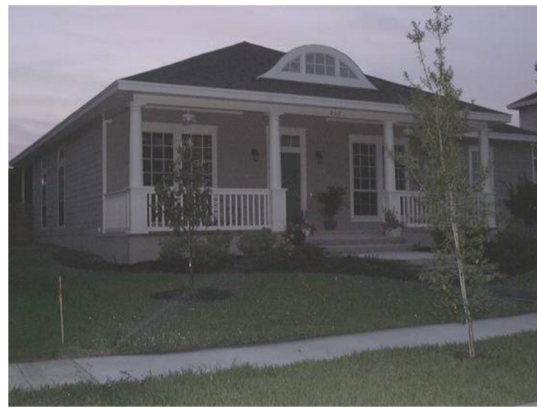
Acceptable: Good roof detailing, adequate porch size and design.
