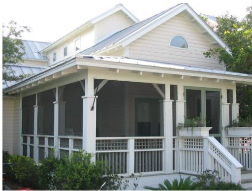
Acceptable: Front porch sufficiently large, adequate column design, interesting hand rails and rooflines.
