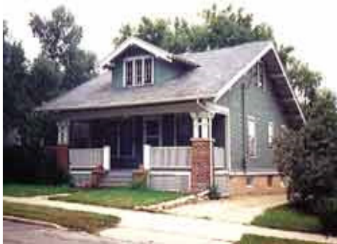
Acceptable: Large front porch, raised foundation, unique dormer, deep roof overhangs, good use of brick and acceptable color scheme.
