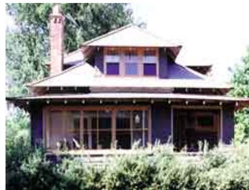
Unacceptable: Front porch enclosed and color scheme, however the raised foundation and interesting roof lines are acceptable.
