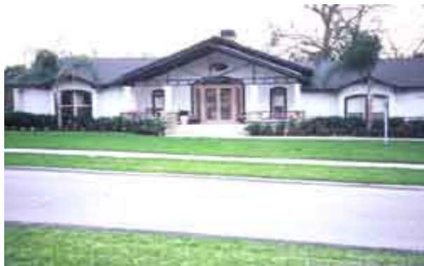
Unacceptable: Small front porch, typical ranch style roofline and lacking in sufficient character.
