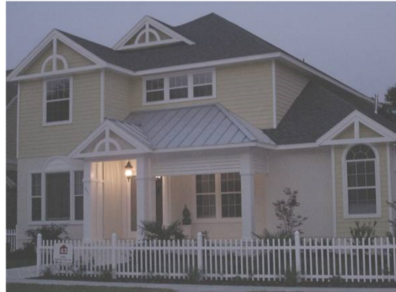
Unacceptable: Front porch too small and foundation height insufficient.
